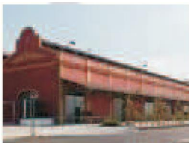
PIER MAUA S/A
